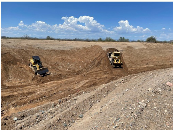
Two dozers work to shape the guide banks of the new Agua Fria River Bridge.
