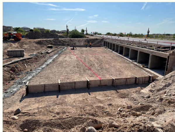
Workers set concrete forms for the floor of the McMicken Dam Outlet Wash Box Culvert.
