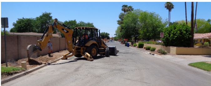
Construction at Gilbert & Hackmore 2018 SPAP Project
